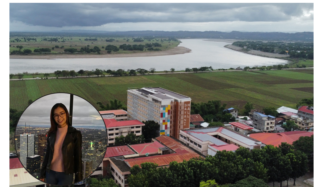
Photo inset: Bayani Hall Lecaros investor Arolyn Madrid. Bayani Hall Lecaros is now operating and is currently being managed by CURA Property Management.
