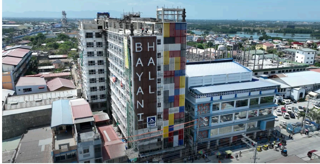
Photo: Bayani Hall Dagupan on-going exterior finishing and interior construction.
